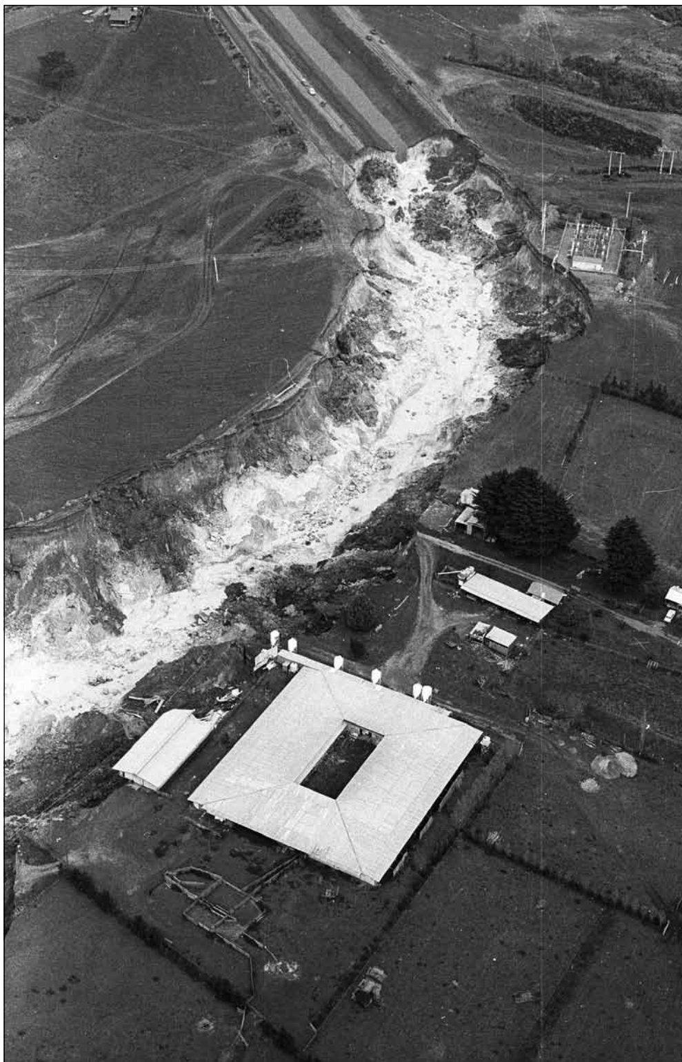
Figure 7.10: The Ruahihi Canal immediately after its collapse, 21 September 1981 Photographer unknown. Reproduced courtesy of Bay of Plenty Times (FO108).
