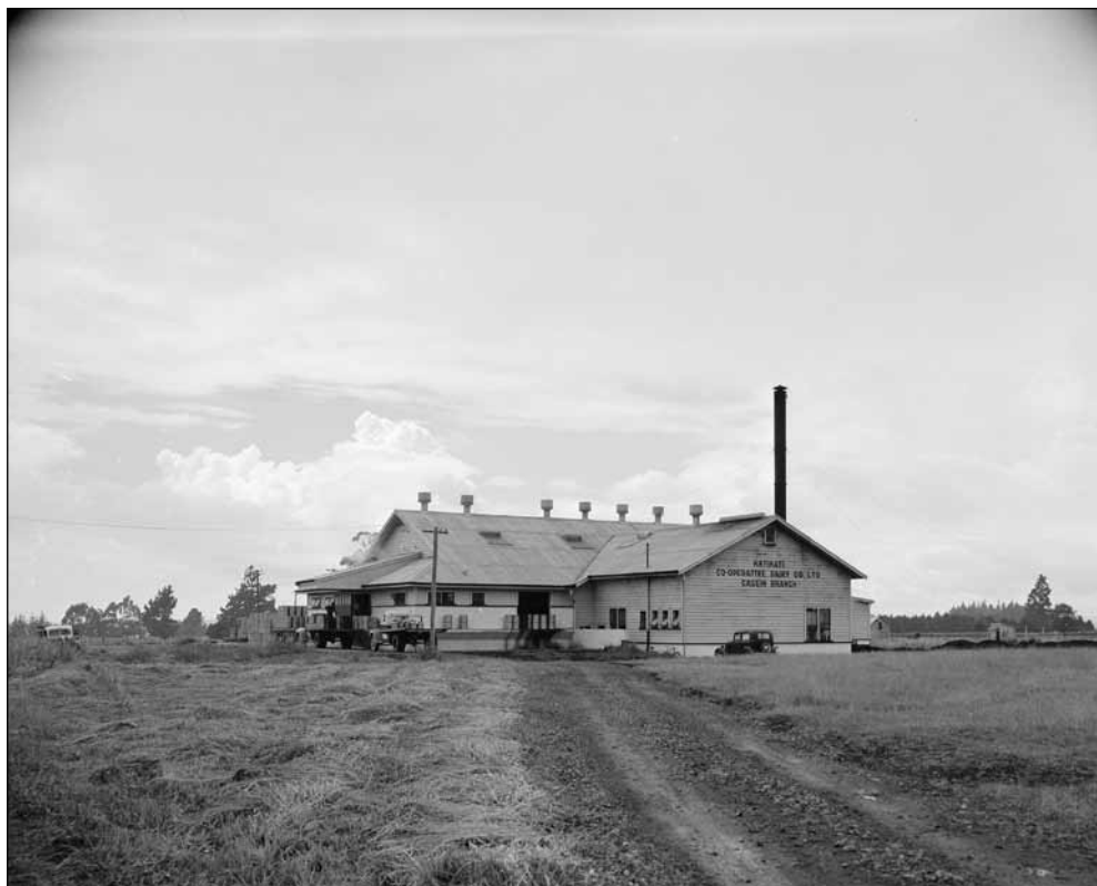
Figure 7.11: Katikati Co-operative Dairy Company factory, 1948
